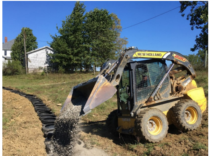
Figure 5. The tread cylinders are filled with rock.
