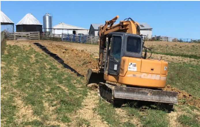
Figure 3. A backhoe creates a trench for the all-weather path.
