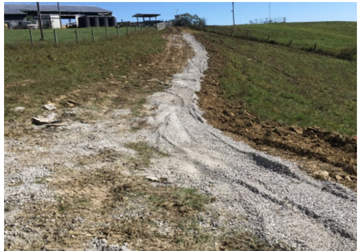
Figure 6. A completed trail leads to a water source located on a hill with 30-percent slopes.
